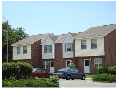
Renovation of Lassiter Courts is made possible through the federal Rental Assistance Demonstration (RAD) program. Work will start late spring.
