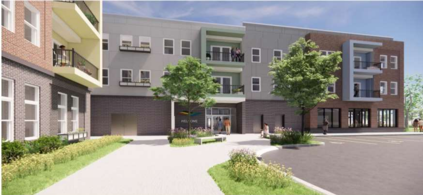
PARKING LOT ENTRY
